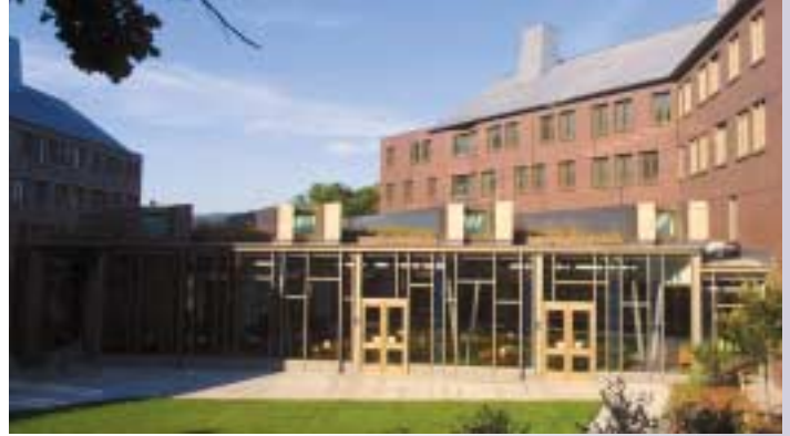
Throughout the course of the project, construction crews had to maintain the bed count while adding new space. Students moved into the first phase of the project, the Alice H. Cook House, in August 2004.
